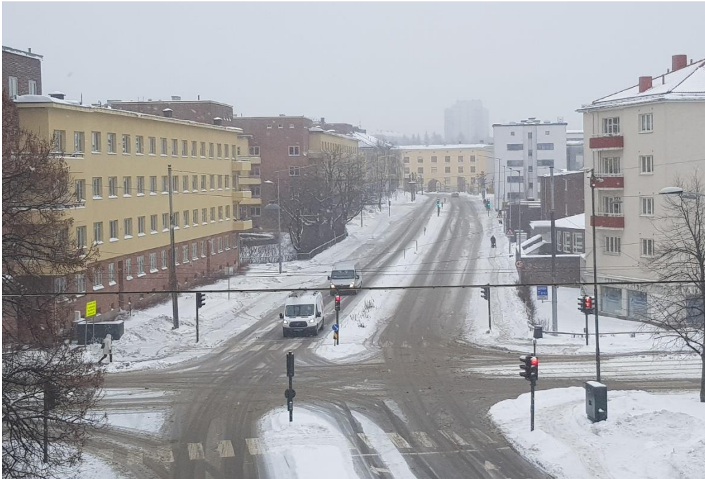
Figure 10. View from the transmitter's side.
